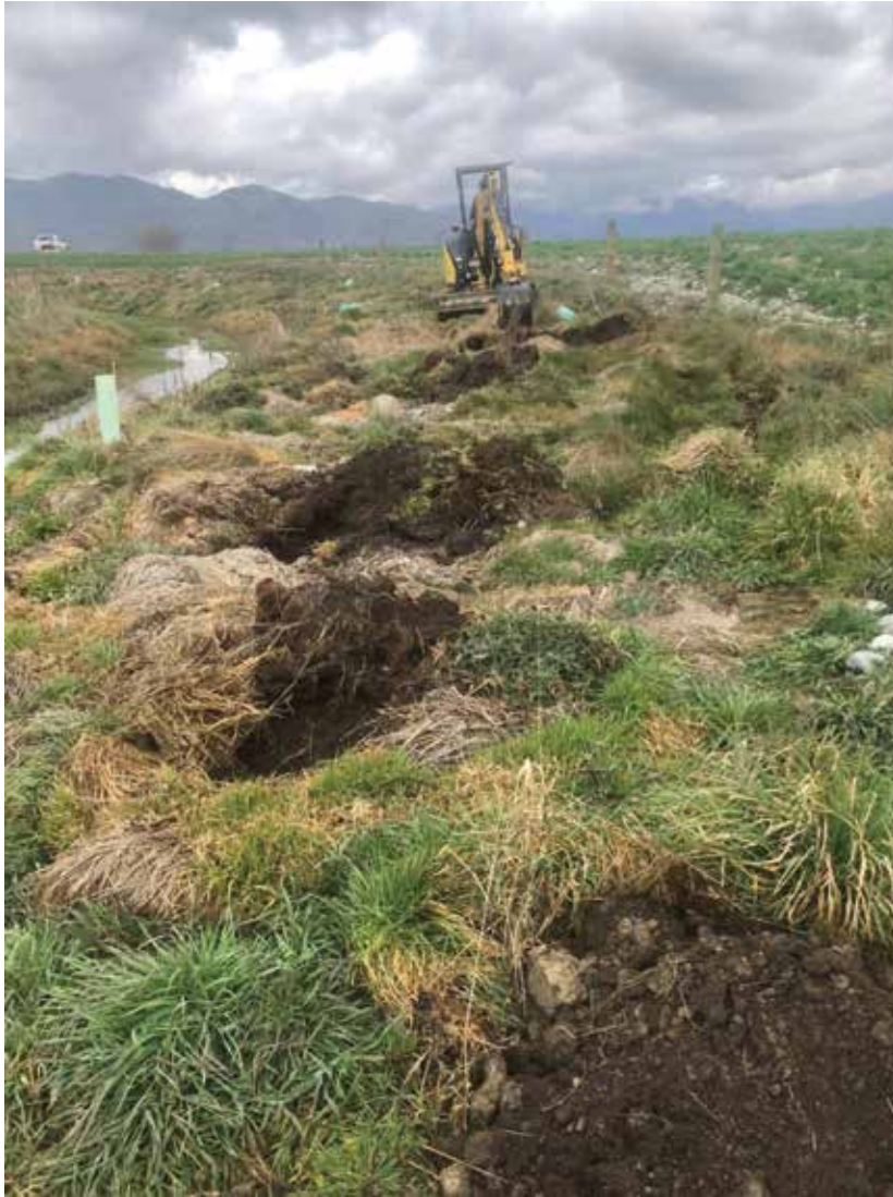
Figure 5-3. Digging planting holes with a small excavator, Omarama Station.
